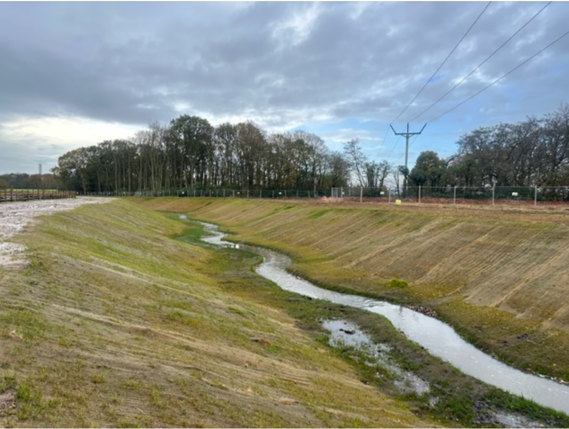
Further views of river diversion works.
